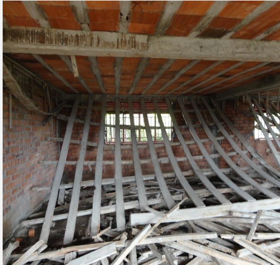
FORMWORK REMOVAL
