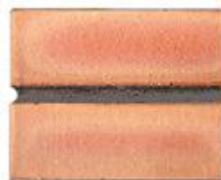
Rolled Joint
